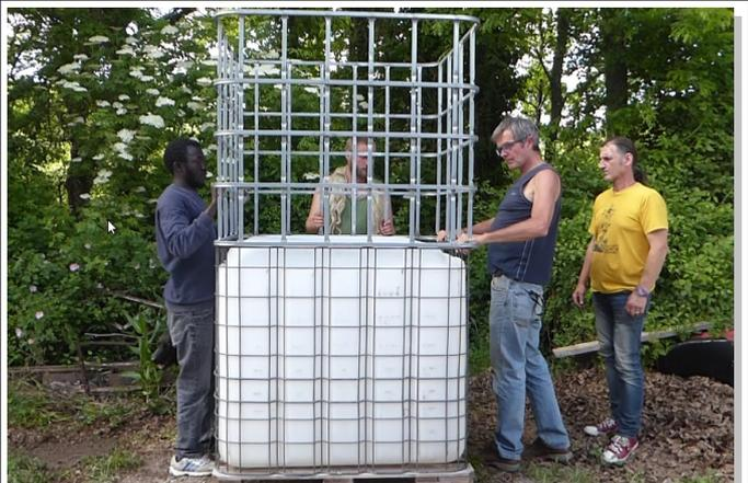
Then put the second cage on the top of the lower and fix it with cable stripper or pipe clamps.
