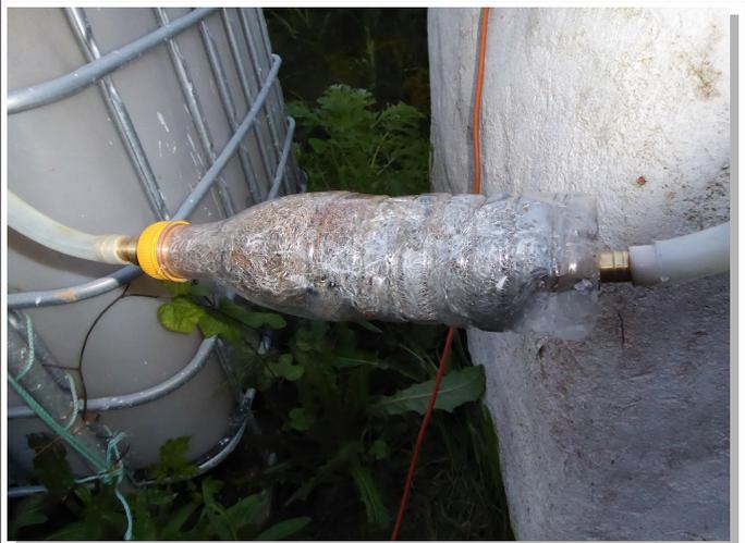
Connect the gas outlet of the digester with the in/outlet of the floating drum. *OPTIONAL* you can add a bottle with iron sponges (not stainless) in the pipe to remove the sulphur.
