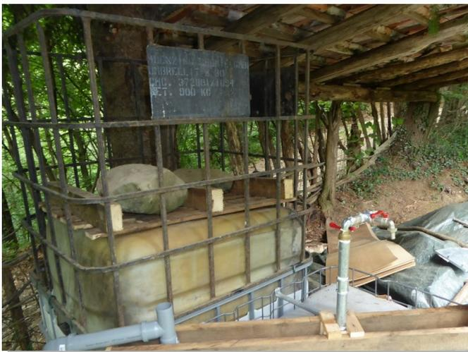
Use a pallet on top of the upper IBC. Give some weight, with sand bags or stones to have some pressure in the gas storage. 10Kg on 1m<sup>2</sup> give you 1mbar; 150kg/m<sup>2</sup>=15mbar, that's a good pressure!
