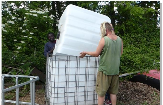
Upper IBC(floating drum): Lift the second IBC out of its metal cage. Open one side of the container for the water in/outlet. Cut it also a bit shorter (~3") to fit better into the lower IBC. Test if the upper IBC slides into the lower IBC easily. If you still feel tension cut a little more of the sides.
