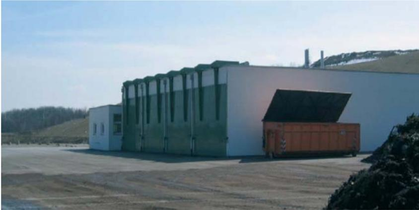
Figure 4.48 Four big size bioreactors for batch dry fermentation.<sup>87)</sup>
